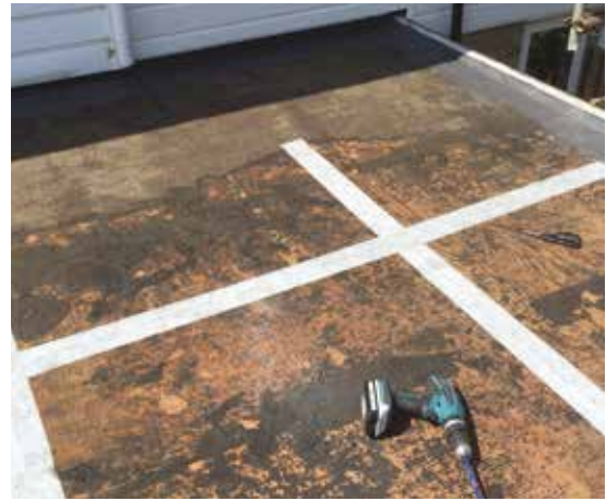
Prepare the surface: Use jointing tape to cover joins in the surface
