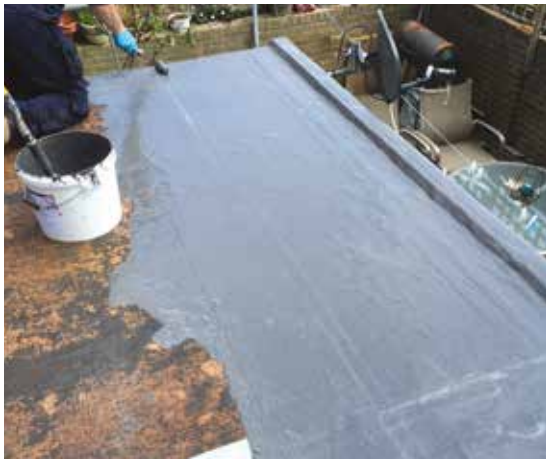
Apply FIX-R Liquid Waterproofing
