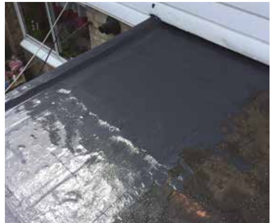
Apply FIX-R Fabric to reinforce
