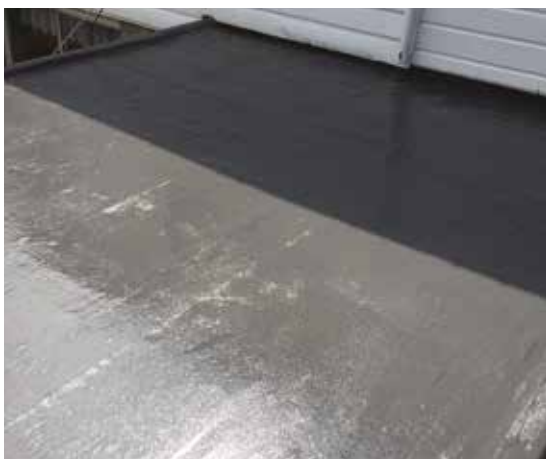
Apply a further coat ensuring 1.5L/m 2 coverage to finish the roof.
