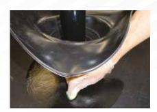
2 Once in position clamp the seal to the pipe with the supplied metal clamp and mark around the base of the seal to give a line to prime up to. Pull pipe seal upwards on pipe to expose the membrane and apply Fix-R EPDM Primer to the EPDM deck membrane.
