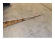
1 Ensure there is no gap between the membrane when butt jointing. The 152mm tape should be centrally located over the joint.
