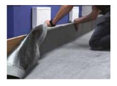
**3** Applying positive pressure to the membrane work the membrane up the upstand to the desired height. These areas should be rolled to achieve a strong bond between membrane and substrate.
