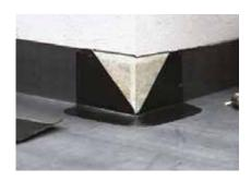
2 Apply Fix-R EPDM Primer to the marked area to be taped and allow to dry. The area must be clean and dry before application of primer, apply primer to membrane and to upstand substrate. Fix-R EPDM Primer must be allowed to dry before application of tapes.
