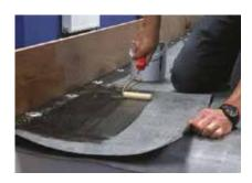
1 Apply Bonding Adhesive to both substrate and reverse of the Fix-R EPDM membrane.
