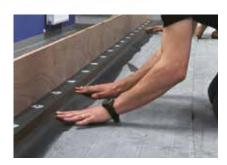
**3** Once the primer is dry remove the protective strip from the PS tape on the RUSS. Guide primed membrane onto the PS tape. Avoid wrinkles or air pockets. Smooth by hand then roll with hand roller.
