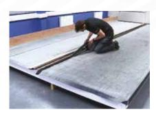
2 Using moderate pressure set the Seam Tape into place to keep air from being trapped under the tape. Unroll the 76mm PS Tape along the length of the seam, aligning the tape (not the clear backing) along the chalk line. Care must be taken not to get any bubbles or wrinkles in the tape.
