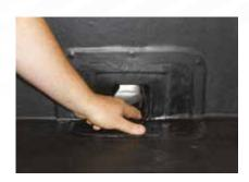
2 Install 228mm PS Uncured Flashing to the outlet. This should be large enough to join onto the membrane by a minimum of 50mm. Cut a 30mm diameter circle from the middle of the tape. Mould the tape into the outlet pipe. Cut a second section of Uncured Flashing 100mm wide. Prime pipe and apply this to outlet.
