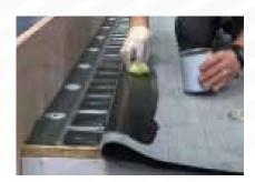
**2** Apply Fix-R EPDM Primer to target area on the underside of the EPDM membrane that will come into contact with the 76mm PS tape on the RUSS.
