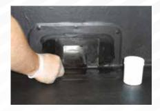
1 Install outlet into parapet wall before installing EPDM membrane. Install Fix-R EPDM membrane over the outlet with Fix-R EPDM Bonding Adhesive. Cut the membrane away from outlet opening by 25mm. Apply Fix-R EPDM Primer to the membrane, outlet face and into the outlet pipe.
