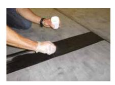
**2** Apply Fix-R EPDM Primer to the area to be seamed. Apply primer 80-100mm either side of the join of the EPDM sheets.
