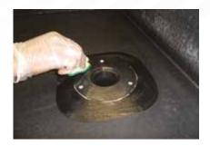
1 Cut the outlet flange back to leave a min. 50mm to deck. Cut the membrane back to meet the perimeter of the outlet head. Secure the outlet to the decking and apply Fix-R EPDM Primer to the head of the outlet and to the EPDM membrane.
