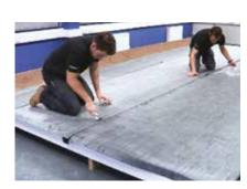
3 Lay the top membrane onto the Seam Tape. Pull away the clear backing from the tape at 45° degrees to the seam. While removing the poly backing, apply pressure across the seam, from the back to the leading edge. Roll the seam at right angles to the seam direction, & along it.
