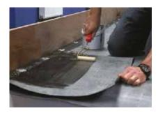
**4** Once secured to the RUSS finish the upstand by using Bonding Adhesive to the remainder of RUSS, upstand and membrane.
