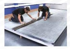
1 Fold the top sheet back to expose the seam area. Using a scrubbing pad apply the Fix-R EPDM Primer to the seam area. Apply the primer past the seam edge to the line. Fix-R EPDM Primer must be dry before application of PS tapes.
