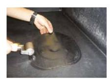
2 Apply the 228mm PS Uncured Flashing to the primed area. Once fitted cut a small section from the centre of the tape out to expose the outlet opening and press the remaining tape down into the outlet. Roll the entire flashing with a 50mm hand roller.
