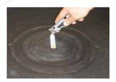
1 Fit the outlet into the roof before installing the membrane; ensure the outlet has the yellow protective cap installed. Install the Fix-R EPDM membrane to the roof and over the outlet. Place cutting guide over the pin and cut round the circular plate.
