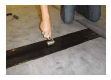
**4** Once the entire length of tape is applied to the seam, roll across the 152mm tape with hand roller. Where 152mm tapes intersect other tapes, 228mm PS Uncured Flashing cover patches must be applied.
