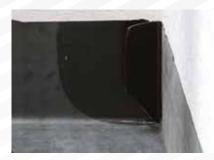
1 Form excess membrane into neat flap. Cut back to leave a 76mm wide flap. Apply Fix-R EPDM Primer to the front & back of the flap and to the membrane on the wall. Fix-R EPDM Primer must be allowed to dry before application of PS tape.
