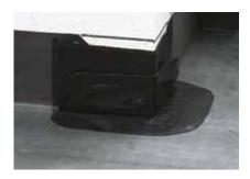
**3** Start installing the tape from the top point. Work the tape down upstands first and into the bottom angle change.
