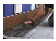
2 Once the adhesive has become touch dry with no wet puddles, mate the two surfaces together. Leave no voids between the Fix-R EPDM membrane and the receiving surface.
