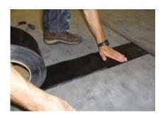
**3** Once the Fix-R EPDM Primer has dried, peel back 150mm of the poly backing and press the PS tape into the primed area. Once the tape is held in position, peel back the poly backing and smooth the tape into the primed area. Progress along the seam.
