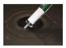
3 Insert a bead of Fix-R EPDM Water Cut Off mastic between the underside of the membrane and the top flange on the outlet. Screw in the clamping ring till it's completely tightened. Use the two tightening lugs to apply leverage to the ring.
