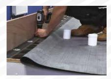
1 Mechanically fasten RUSS to decking or vertical upstand at 300mm centres. The PS section must face main field area.
