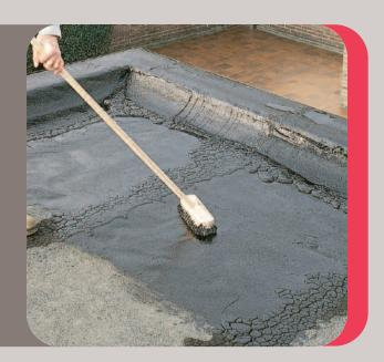
TO PREPARE AND STABILISE SURFACES PRIOR TO APPLYING ROOFING FELT AND FLASHING TAPES.
